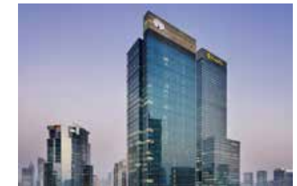
JING AN KERRY CENTRE Shanghai
